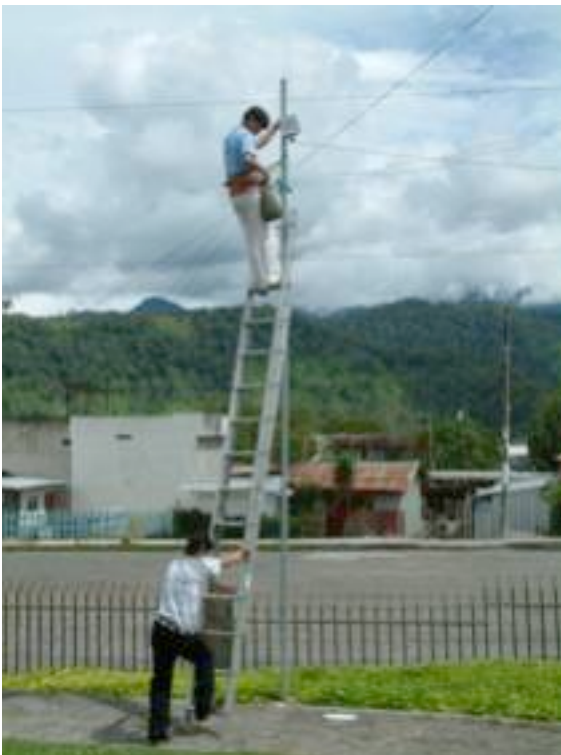
Local technicians during installation.
