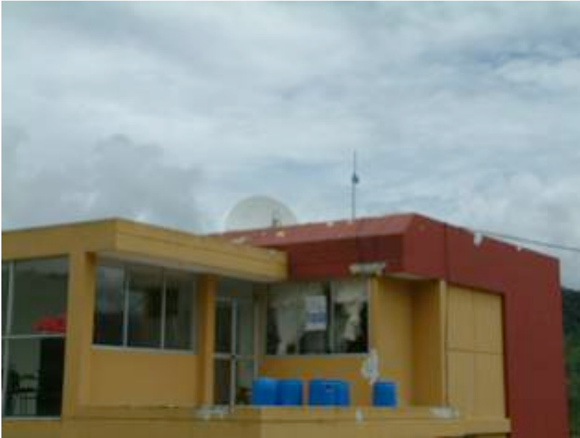
Health Station with VSAT and Wi-Fi Antennas
