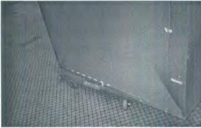
Figure 5. Damage to a map cabinet. Photo-document all problems to substantiate later claims.
