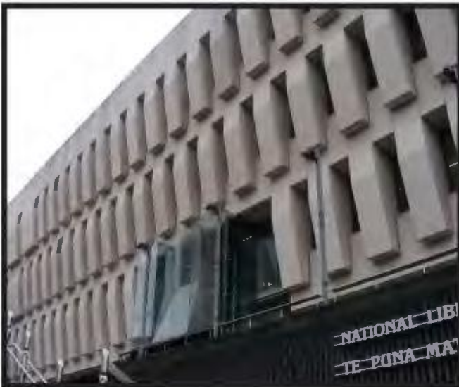
Figure 24- Te Puna Building
