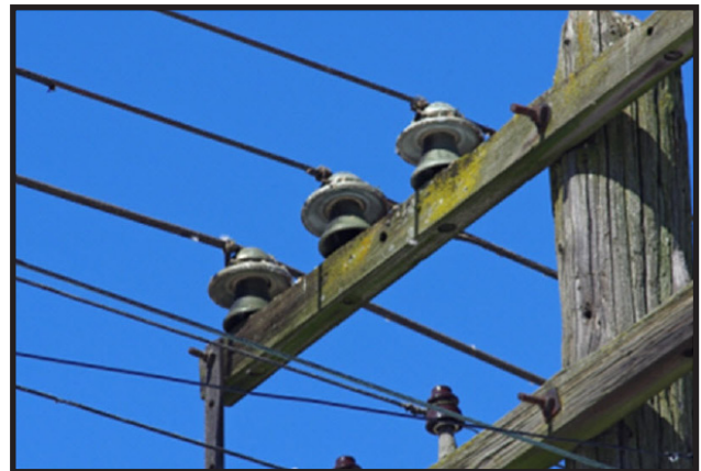
Three Thomas M-2255s remain in service for well over 100 years on Toronto's antiquated downtown street side distribution lines.
