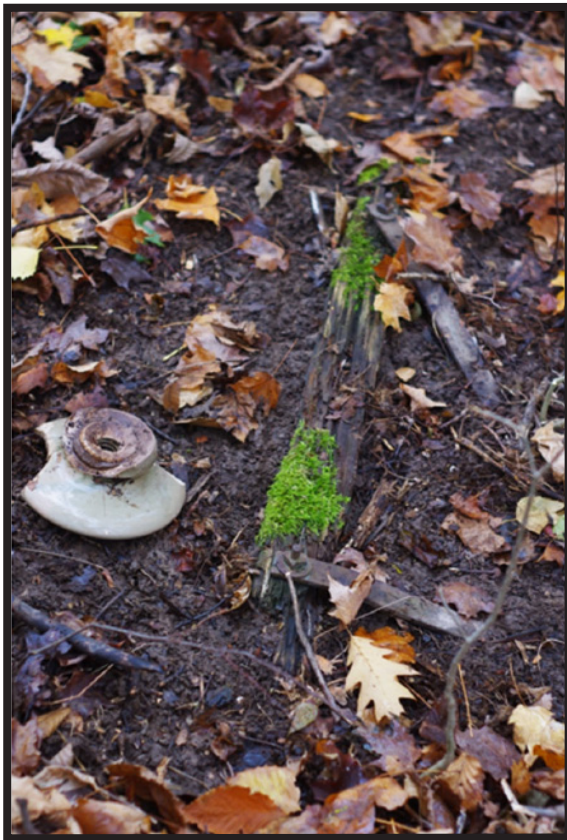
Remains from of an original pole site with cross-arm and broken insulator on the Tile Works line referenced in the text.
