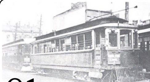
Image courtesy of Ontario Hydro
