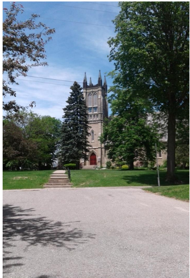
Figure 2 - St. James Anglican Church
