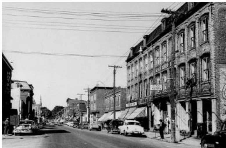
Figure 2. Original Main Street Morrisburg 1950's
